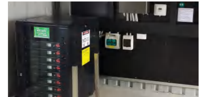
Rack-mounted lithium battery
